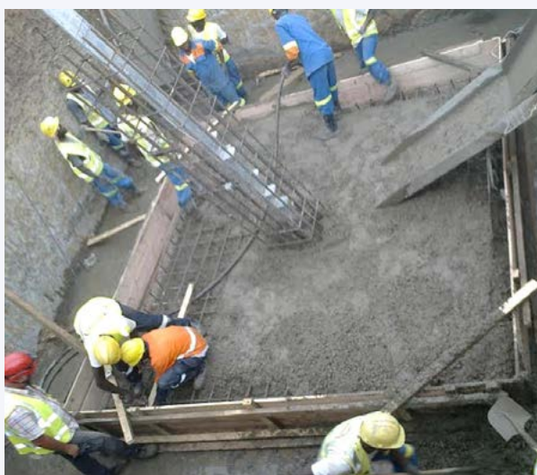
Interconnection Project. Concreting of Pad March 2015.
