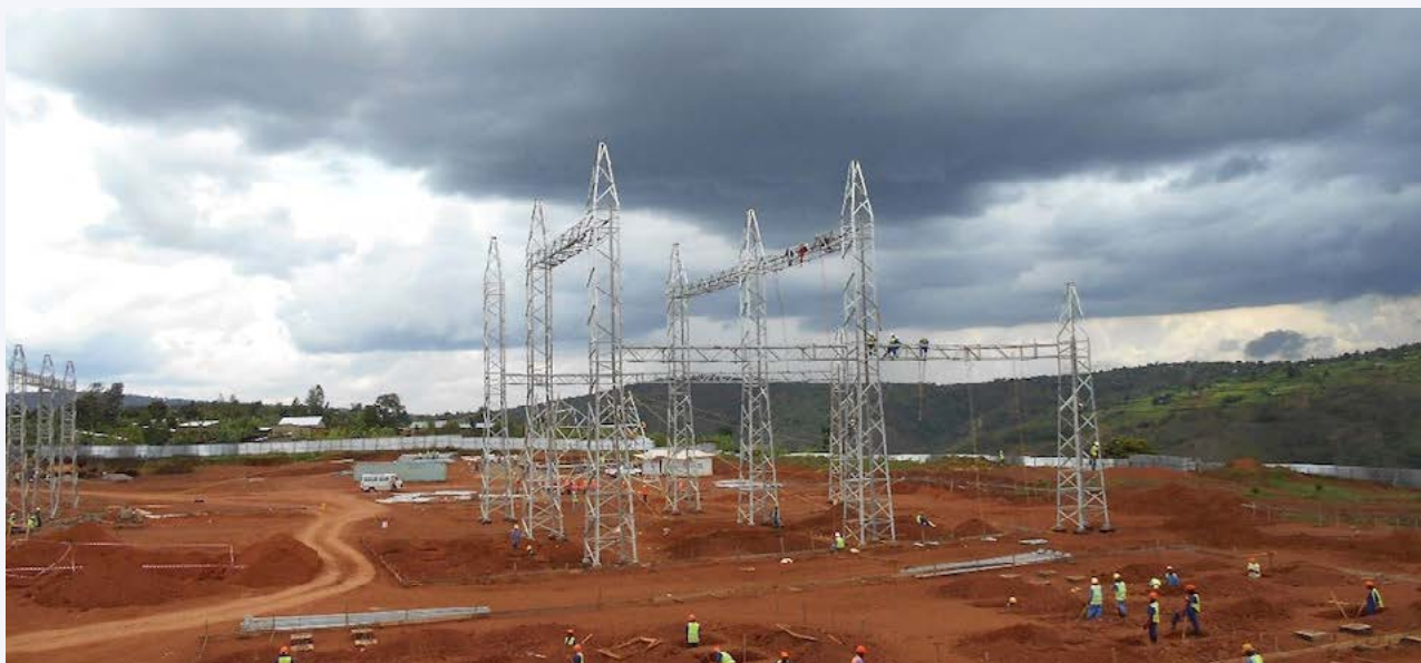
Interconnection Project 220 kV Gantry towers.
